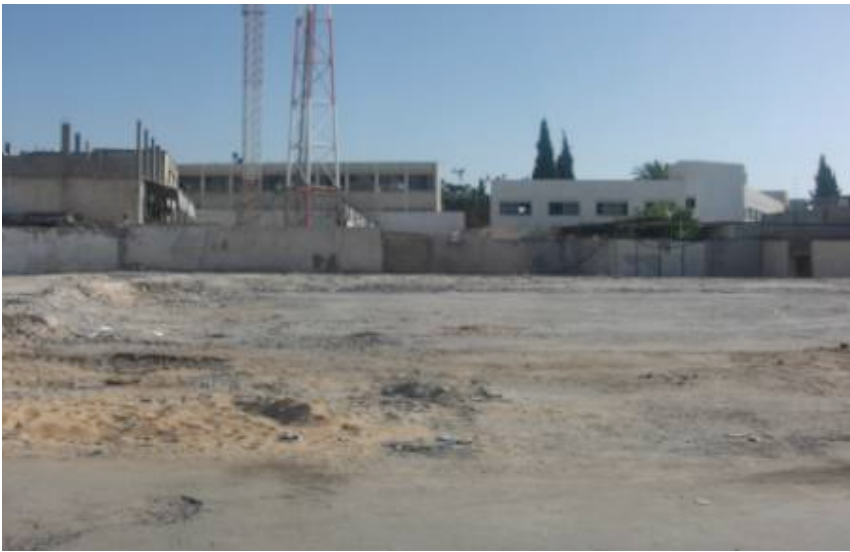
Flattened site of former police station in Deil El Balah
