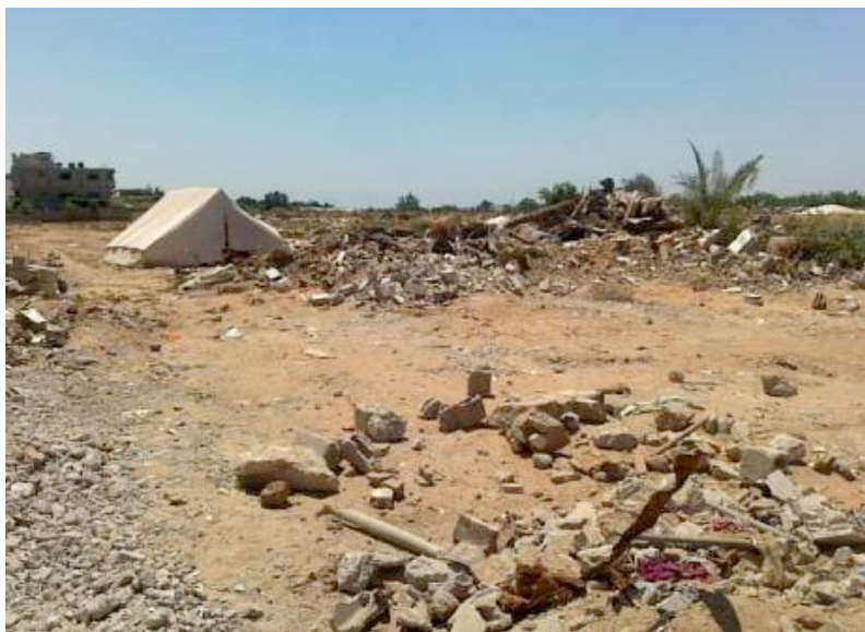
What is left of the El Samouni houses and tent where surviving family live now
