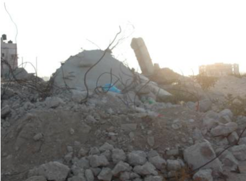
Former home reduced to rubble
