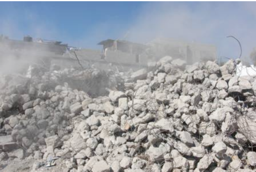
Area where apartment block fell
