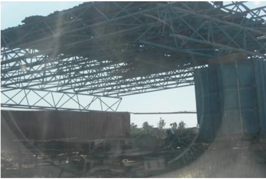
Remnants of another factory
