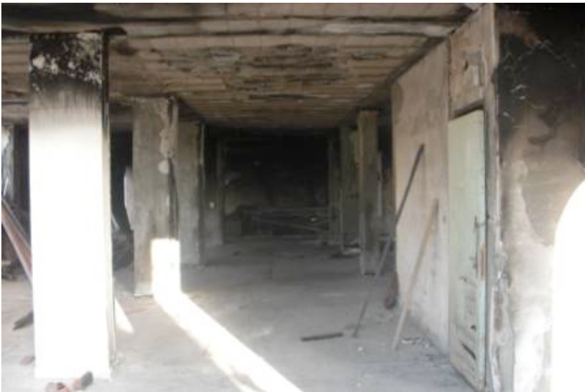
Main foyer of former hospital 6 months on
