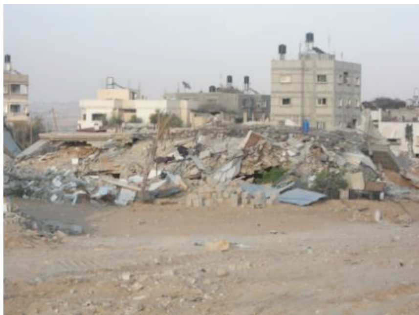
Former home reduced to rubble
