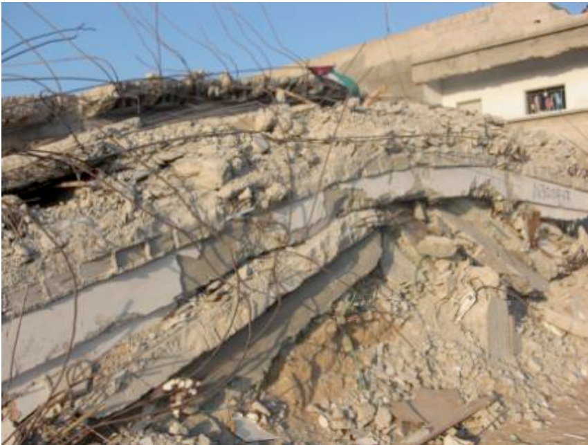
Remains of collapsed home that killed their father
