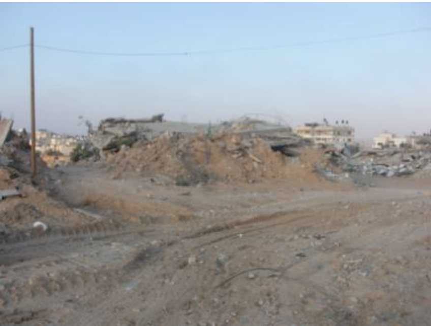
Street of former houses reduced to piles of rubble
